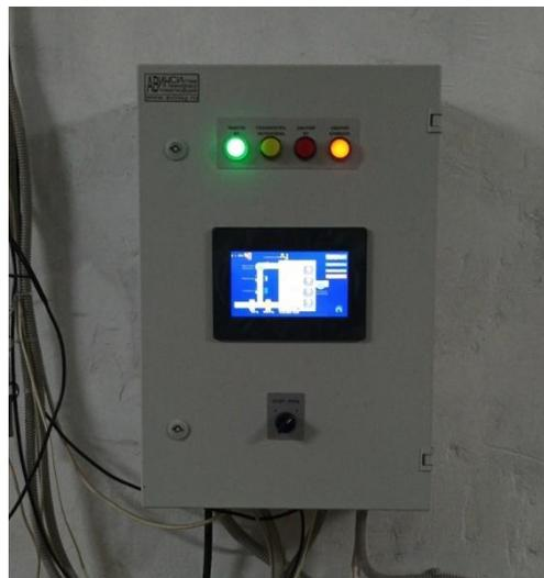
*Figure 2. Cabinet with control computer*
